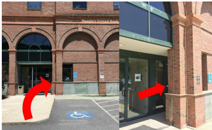
112 State Street, People's United Bank building rear entrance off Taylor Street
